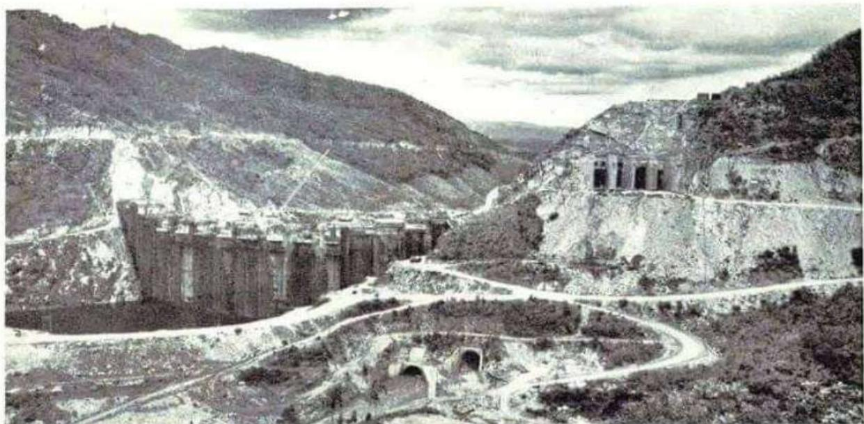
Here is a distant "shot" showing the spillway intake structure where excess water will overflow after the dam is completed.
