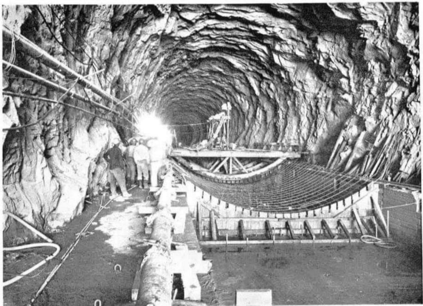
Here we are in the tunnels where the tunnel men are placing concrete with a "Rex" Pumpcrete machine. These men earlier in the job did the excavation of the rock for the tunnels.
